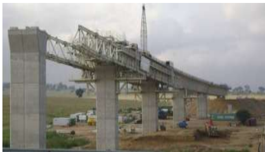
Figure 1 : File photo of viaduct showing launching girders resting on brackets attached to piers
