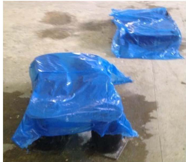
Figure 3: Cylinders Covered in Plastic Sheets for Curing
