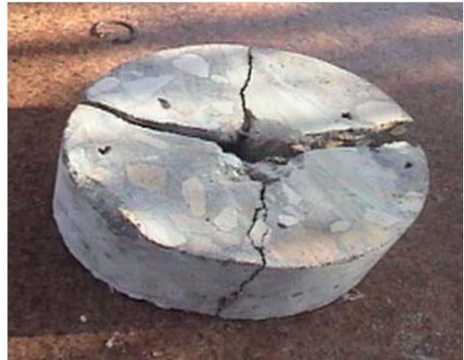
Figure 8: Plain Concrete Impact Failure
