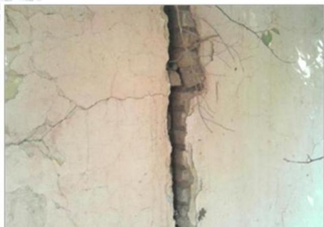
**Damage Category: Severe**. Deep cracks appear in the exterior walls of the building
