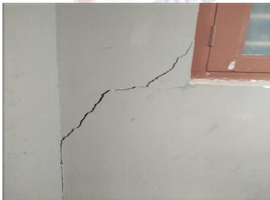
**FIG (3-B) CRACKS IN THE INTERIOR WINDOW WALL**
