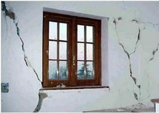
**Damage Category: Very severe.** Serious cracks around window in the interior wall [10]
