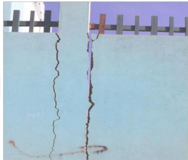
**Damage Category: Severe**, vertical cracks appeared at the joint between column and masonry wall of the fence.
