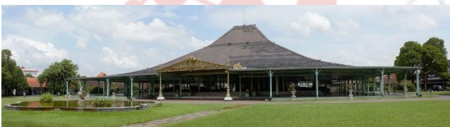
Fig. 19. Exterior of Pendopo Ageng Pura Mangkunegaran. (Wikipedia, 2023).
