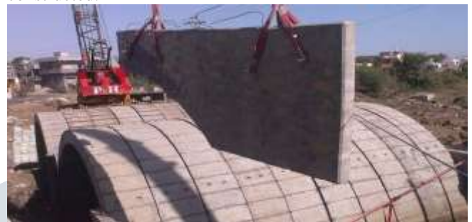
Fig. 7. Installation of Spandrel wall [9]
