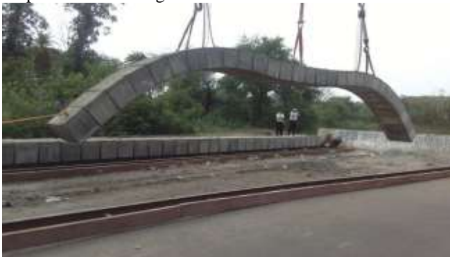
Fig. 5. Half lift of Flexiarch [9]
