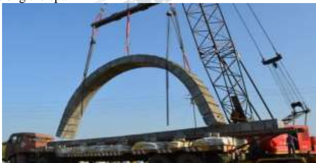
Fig. 6. Full lift of Flexiarch [9]
