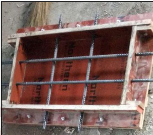
Figure No 2 Mould for casting of specimen
