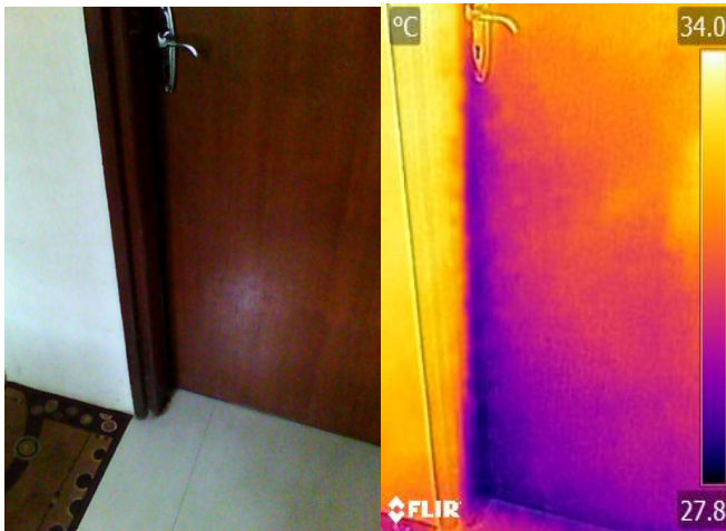
Fig (h): Air leakage through Meeting room
