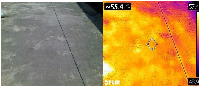
Fig (i): Roof Top at Civil Building
