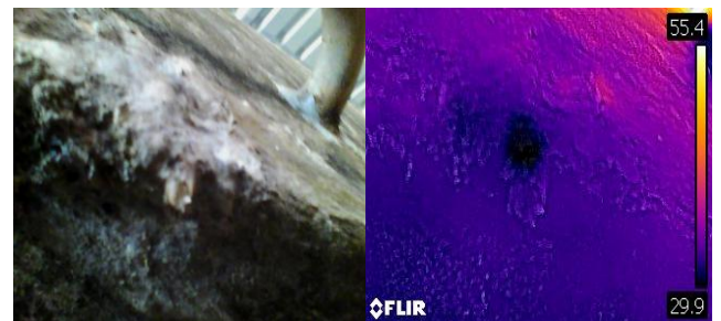
Fig (d): Water Tank no. 24 at terrace (Bottom)
