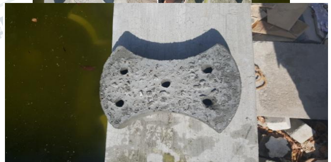
Figure 4 Pavers with holes
