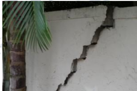
Fig. 1 Damage in shear wall due to uneven settlement.
