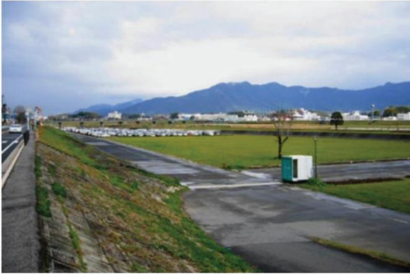
Figure 2. Previous high water channel on the west bank is flat, and a visitor neither feels the longitudinal depth nor sees the water's surface
