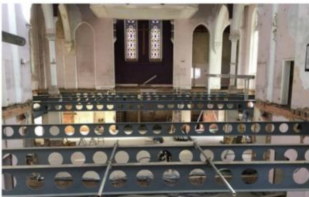
Figure 1: Web openings in beams [12]
