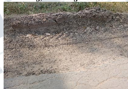
Fig. 8 Heaved lump of soil at the edge of pavement
