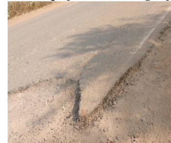
Fig. 9. Edge breaking/Pot holes.
