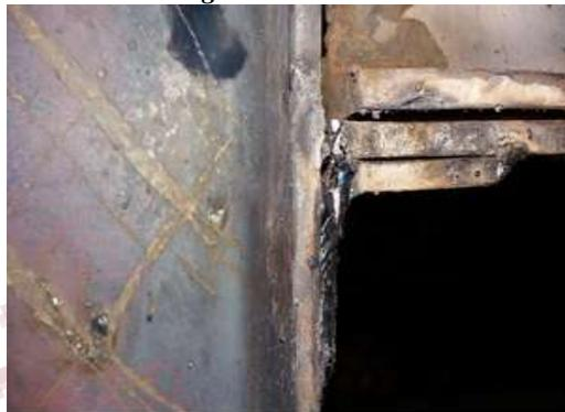
**Fig.5. Failure of moment resisting connection**
