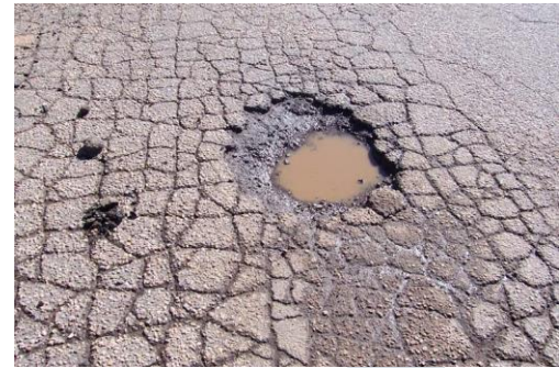
Figure 4.1 (b) Pothole
