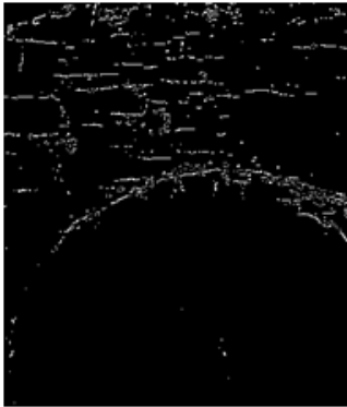
Fig. 13 Cracks obtained by k-Nearest Neighbor
