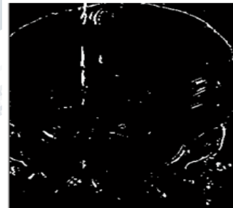
Fig. 3 Cracks obtained by k-Nearest Neighbor
